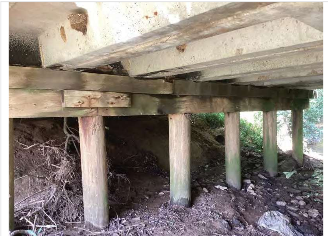
Bent 1 front side
